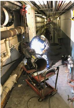
Steamfitter Durante is welding flanges to make final connections in a major repair to the steam-distribution line.
